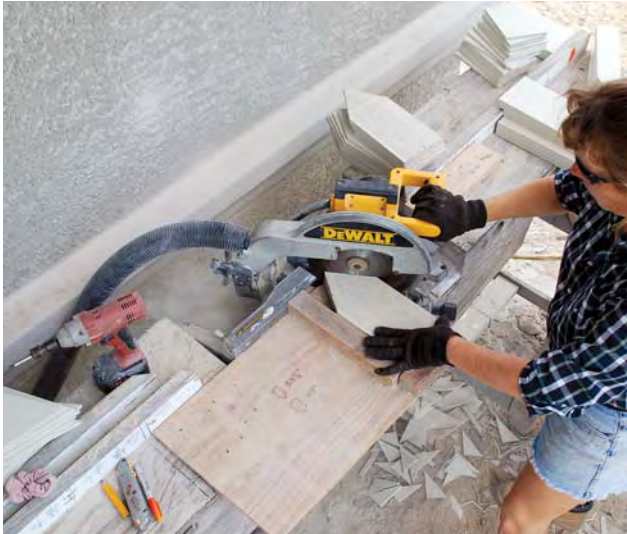
Figure 8. After the blanks are cut to length, shingles are given diamond points and diagonal cuts on the miter saw (left). A simple jig screwed to the saw stand holds a stack of shingles perpendicular to the fence when the angle exceeds the saw's capacity (above).
