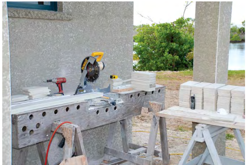
Figure 7. The author's saw stand is sturdy enough to support up to five 12-foot lengths of lap siding — a good 75 pounds of material (above). Stops made from wood scraps can be quickly screwed to the top for repetitive cuts (left).
