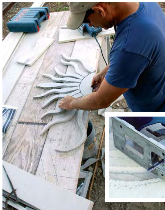
Figure 3. Fiber cement can also be used to make decorative gable treatments. Scroll cuts are made with an orbital jigsaw fitted with a carbide-grit blade.
